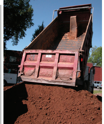
At least six dump trucks unloaded precious soil onto the new garden plot. Each load: approximately 14 tons.
