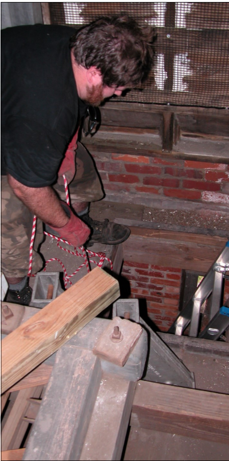
3 Among the toughest chores was hoisting gear more than 30 feet up the bell tower through a narrow entry door to the bell housing. Here, Nathan does the heavy lifting, hauling solid metal up with a rope.
