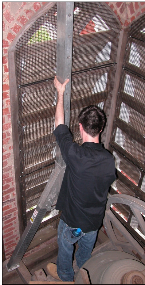
4 Braces were put in place to hold a winch used to lift the bell while the new A-frames were installed. The cramped confines of the bell tower made quite a repair challenge for the two man crew.
