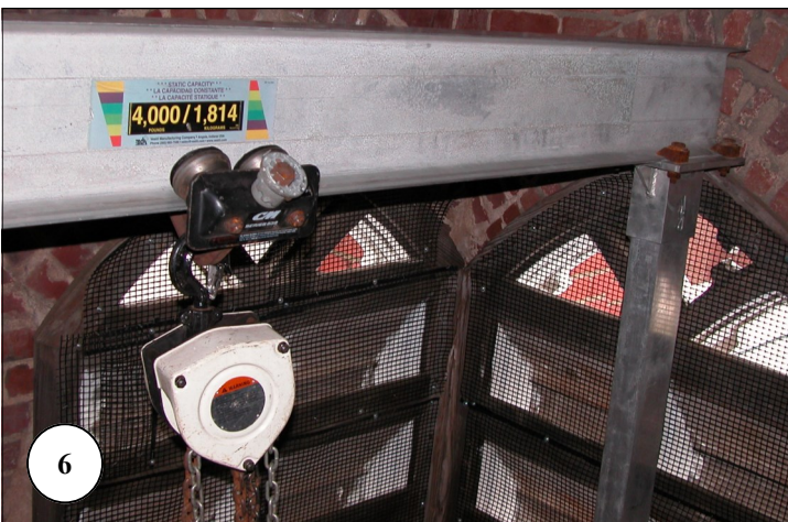
6 The heavy bell needed heavy-duty equipment to lift it into the right position for the new A-frame apparatus. Notice new screens to keep animals out of the belfry.
