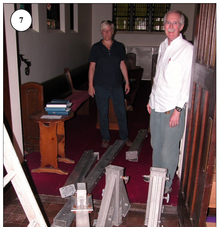
4 Braces were put in place to hold a winch used to lift the bell while the new A-frames were installed. The cramped confines of the bell tower made quite a repair challenge for the two man crew.
