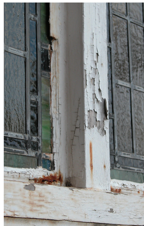
The years and North Carolina weather have taken a toll on our buildings. Repairs to crumbling windows and stained glass are two of more than 20 identified areas of need. Interior portions of the church are in need of attention, too, notably plaster walls and some equipment, among other items.
