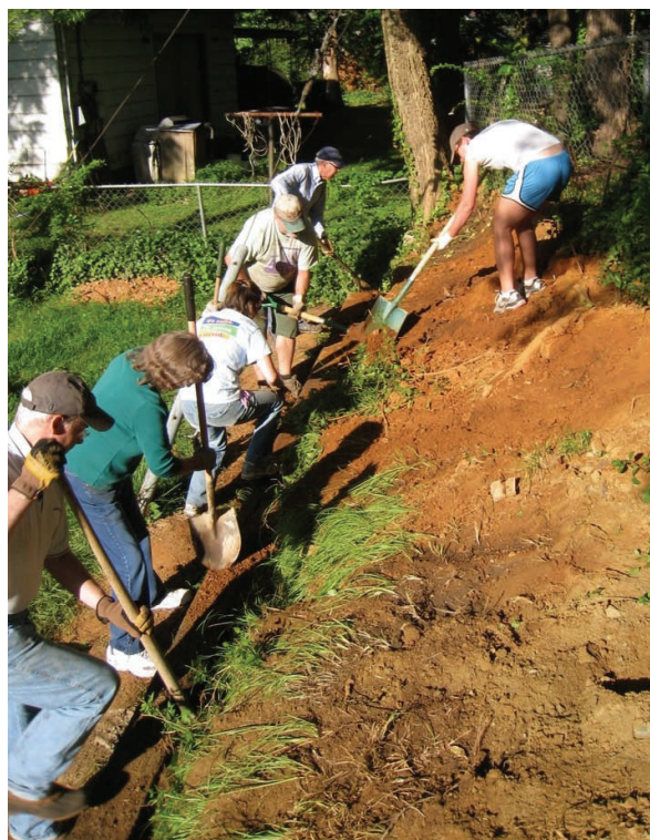
Caldwell volunteers put their shoulders into pushing heavy railroad ties into dense Carolina red clay as they construct an retaining wall as part of a Habitat for Humanity project. Volunteers are welcome - no skills required - on H4H projects.
